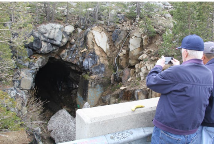
We arrived at Donner Summit and walked out to the historic railroad tunnel from years past.
